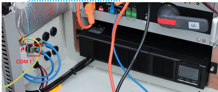
Pic 1.1.6 HV48100 SE cabinet COM 1 port
