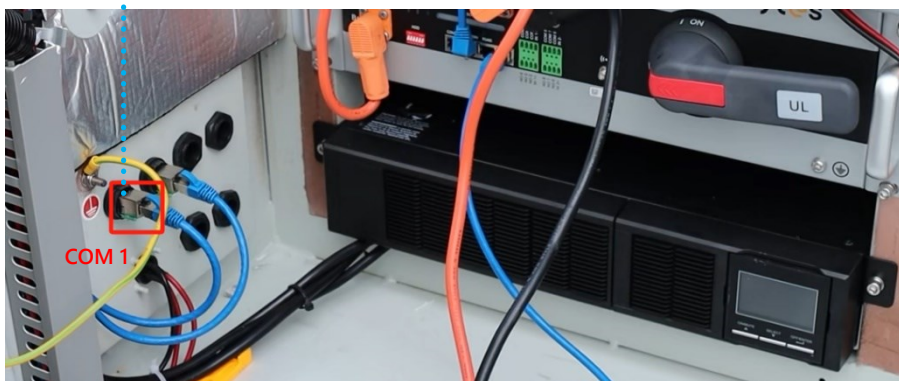
Pic 1.6 HV48100 SE cabinet COM 1 port
